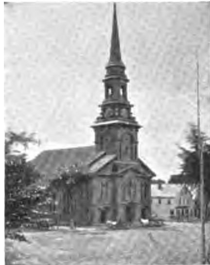
"FROM THE STEEPLE OF THE NORTH CHURCH THE CURFEW IS STILL RUNG AS IN COLONIAL DAYS."
